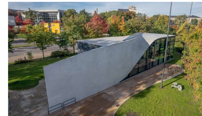
The carbon-reinforced concrete CUBE research building | Stefan Gröschel
