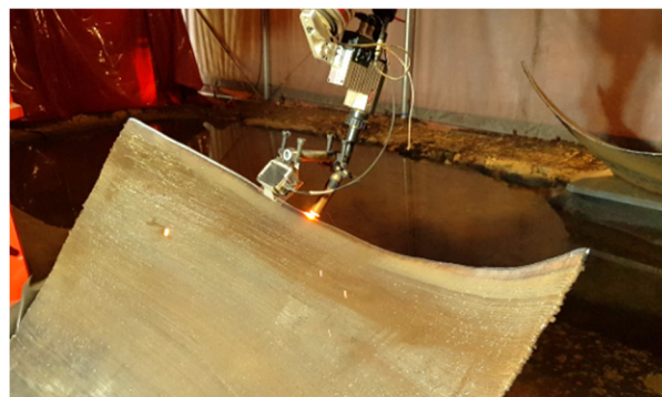
Fig. 2. WAAM printed bridge of TU Darmstadt: during production.
