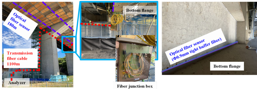
Fig. 3. Optical fiber sensor installation on the viaduct; left: Fiber cable layout from DFOS analyzer to fiber sensor; center: transmission and sensing fibers connected in the fiber junction box installed on the upper deck; right: optical fiber sensor mounted to the top surface of the bottom flange.
