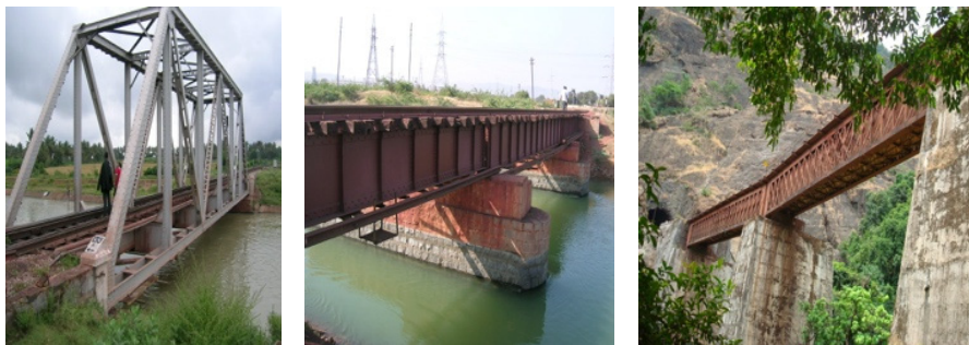
Fig. 1. Bridge 139A, Bridge 3, and Bridge 102, respectively.
